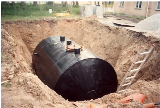
Figure 4 An underground horizontal heat storage tank for a small CHP unit for a multi-family housing area
