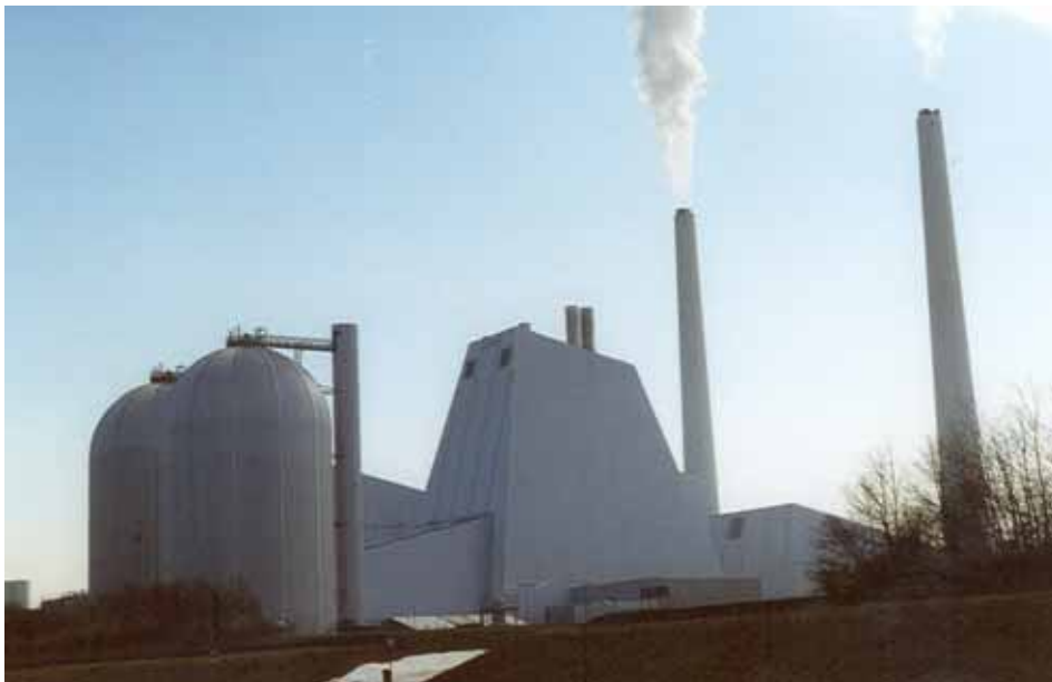
Figure 1 Heat storage tanks in connection with a multi-fuel (Coal, natural gas, oil, wood chips, straw) cogeneration unit, Avedøre Denmark)
