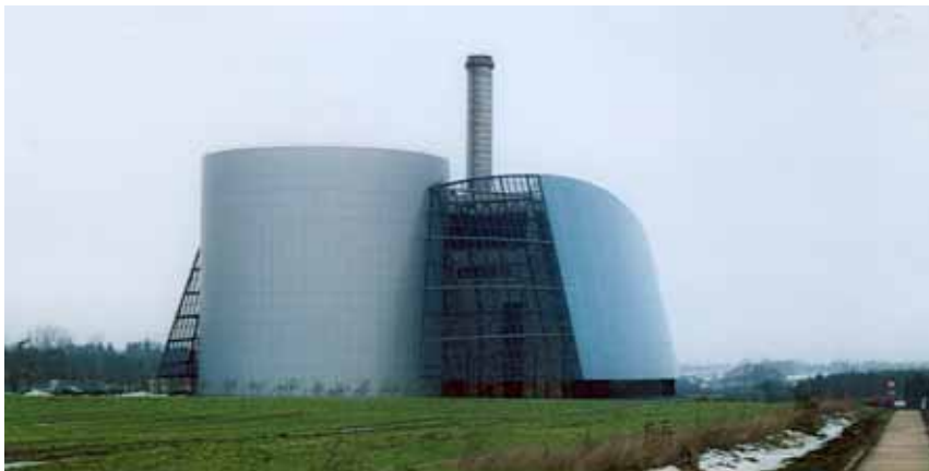
Figure 22 At this gas-turbine based combined-cycle cogen plant the outer shell of the plant hides the heat storage tank from most view angles
