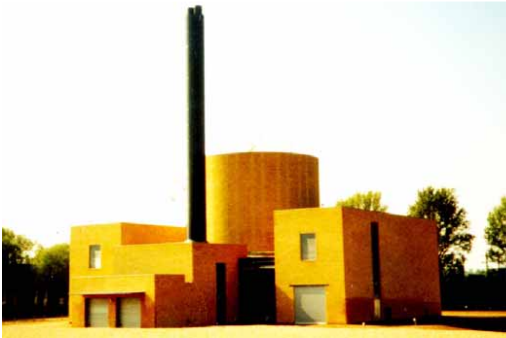
Figure 20 The heat storage tank of this gas-engine based cogen plant has a surrounding brick wall for visual reasons
