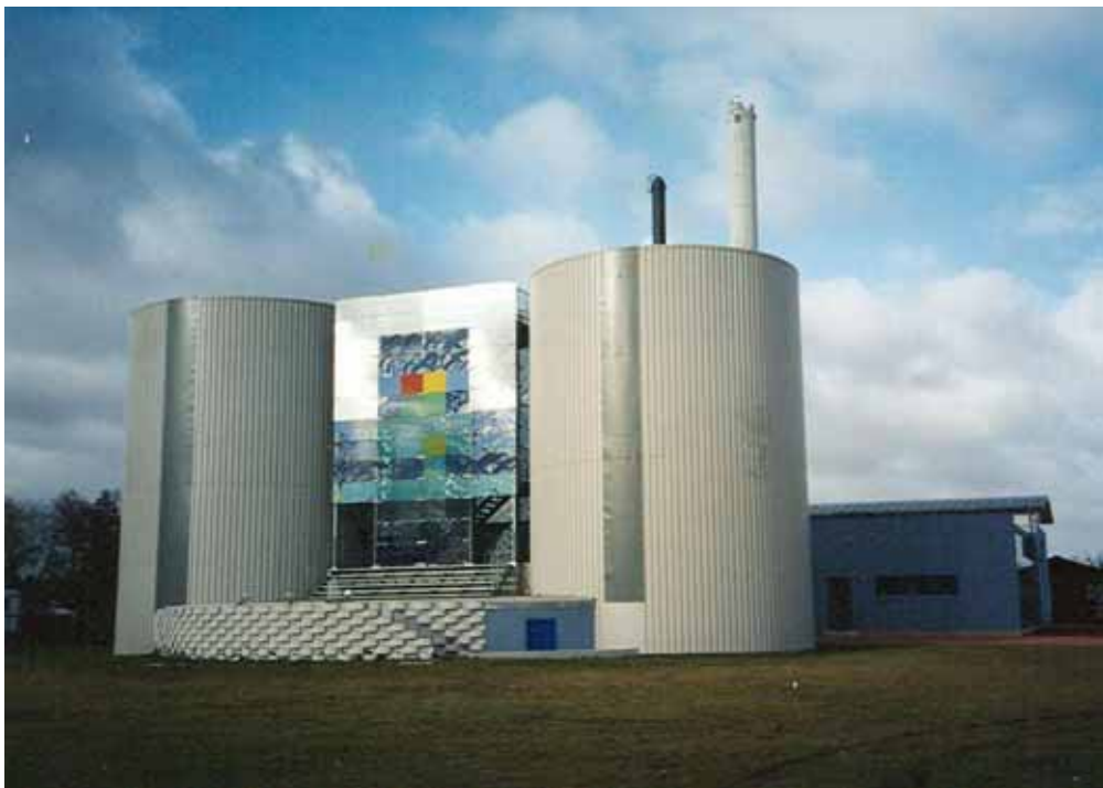
Figure 21 Two vertical tanks framing an outdoor scene erected in connection with a sports ground. A negative attitude amongst locals against such tanks was turned, as this proposal added the outdoor stage and even toilets to be part of the sports ground.
