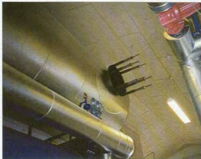
Spring type of explosion relief valve used in exhaust ducting
