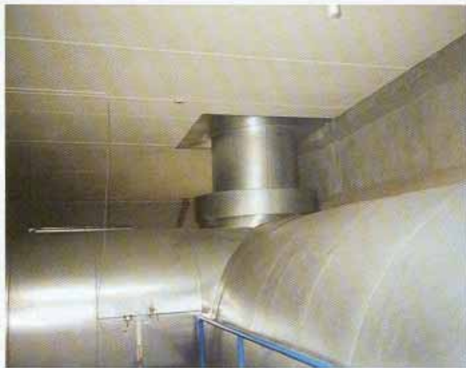
One-off type of explosion relief valve (must be replaced after use)
