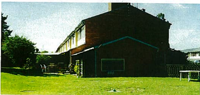
FROM TOP TO BOTTOM: Two vertical tanks frame an outdoor artwork at a sports ground ■ The outer shell of a gas-turbine combined-cycle cogen plant hides a heat storage tank from most angles of view ■ Two underground horizontal heat storage tanks are below this lawn – a few covers can be seen in the grass. The cogeneration unit is in the annex to the house
