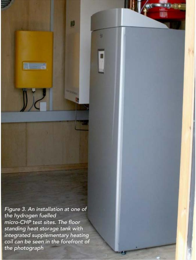
Figure 3. An installation at one of the hydrogen fuelled micro-CHP test sites. The floor standing heat storage tank with integrated supplementary heating coil can be seen in the forefront of the photograph
