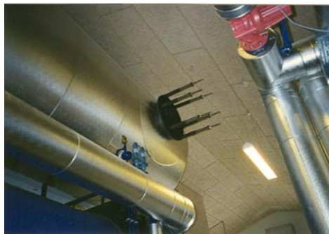
Figure A.2.2: Explosion relief valve, spring type
