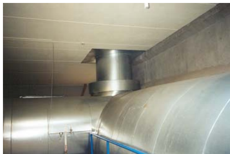
Figure A.2.3: Explosion relief valve, outdoor one-off type
