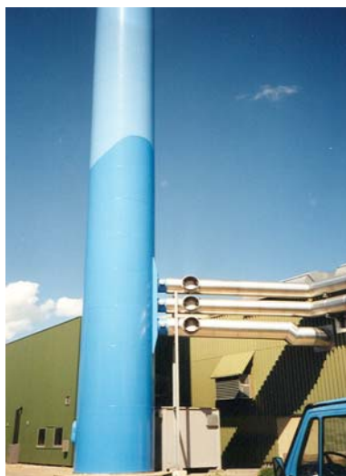
Figure A.2.4: Pressure relief valves to prevent vacuum deformation of thin plate stack tube ducting
