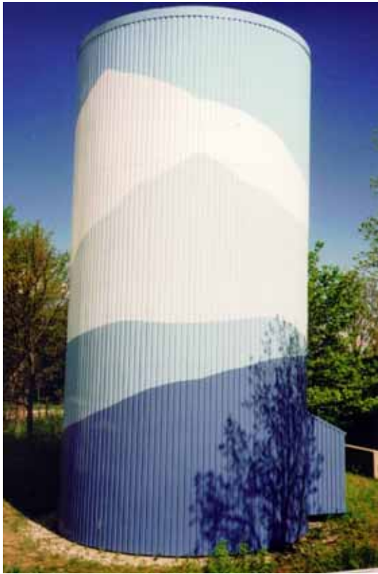
Figure 18 Heat storage tank in art painting
