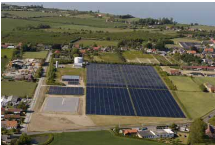
Figure 23 A heat storage tank in connection with a large-scale solar collector (18.000 m 2 ) system; a sand pit storage is used for long term storage (from /8/)
