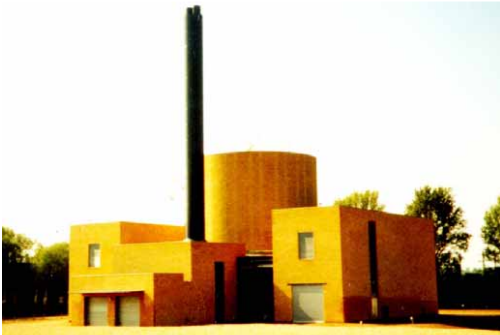
Figure 20 The heat storage tank of this gas-engine based cogen plant has a surrounding brick wall for visual reasons
