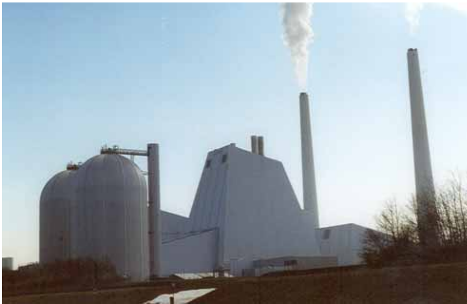
Figure 1 Heat storage tanks in connection with a multi-fuel (Coal, natural gas, oil, wood chips, straw) cogeneration unit, Avedøre Denmark)
