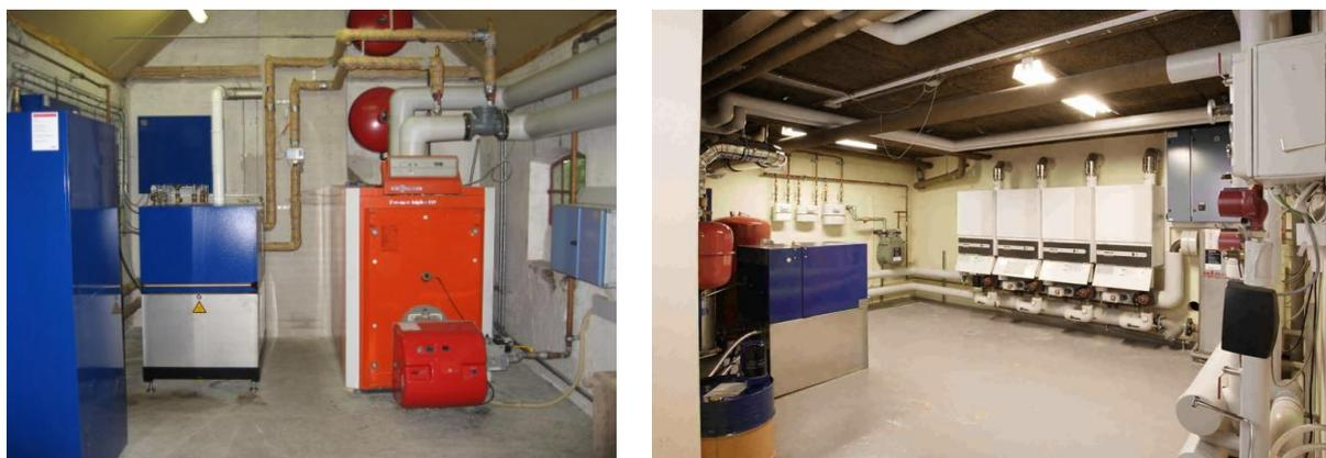
Figure 2 Two examples of a mini CHP unit system (EC-Power) installed in boiler houses
