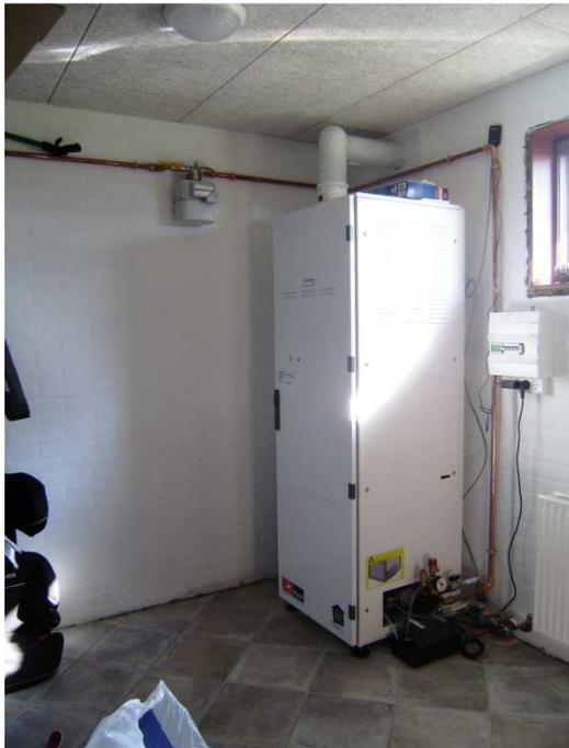
Figure 4: Dantherm natural gas PEM Alpha in phase 3 installed at a field test site.
